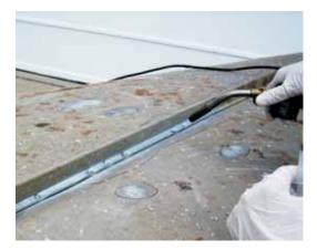
air from the gun. Then, you can either let the G/flex<sup>®</sup> cure at ambient temperature or continue using the heat gun on a lower setting until the epoxy is fully cured.
